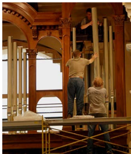
Pedal façade installation
